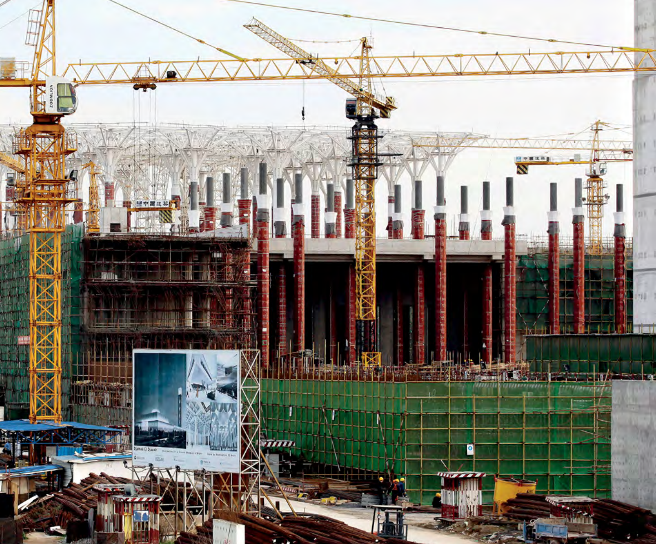
The new Great Mosque in Algiers, being built by the China State Construction Engineering Corporation (January 2016).
