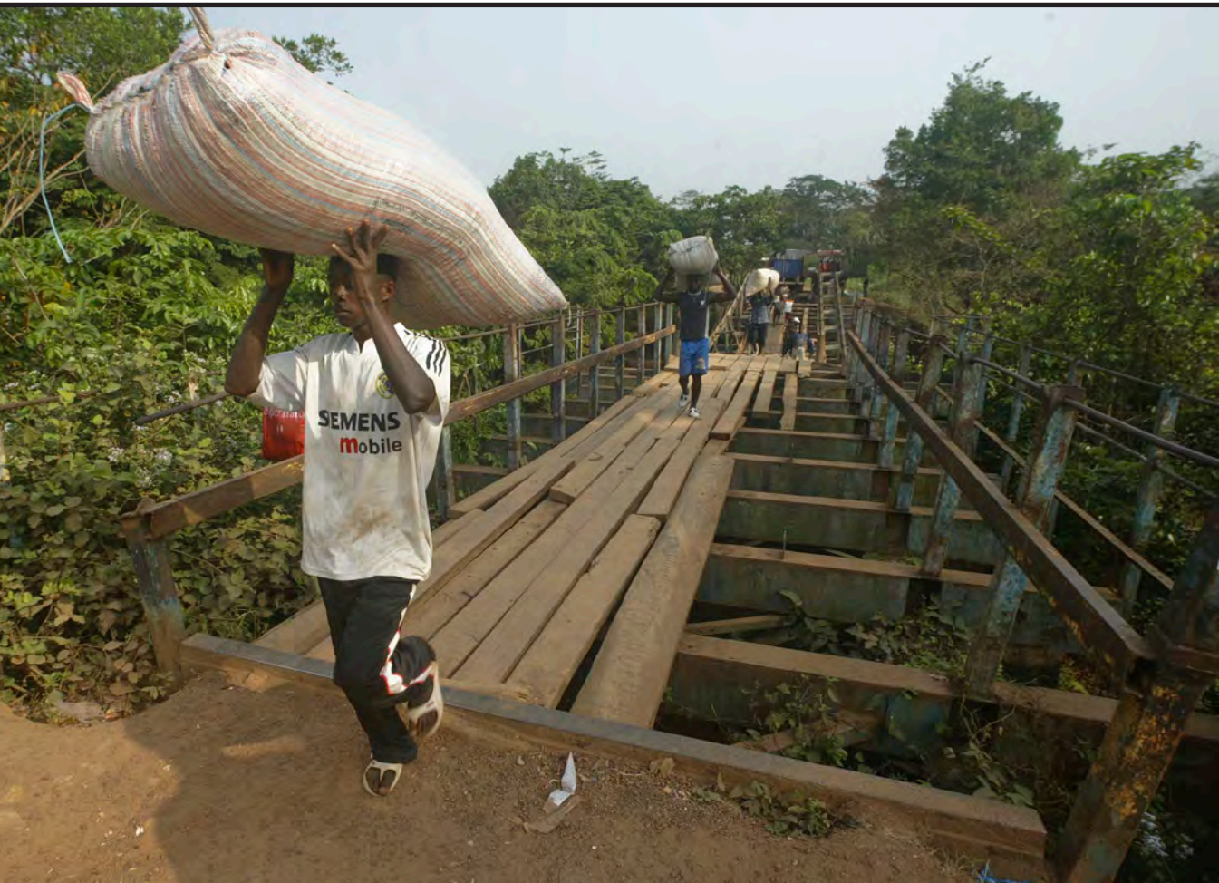
Bridge infrastructure, Ivory Coast into Liberia
