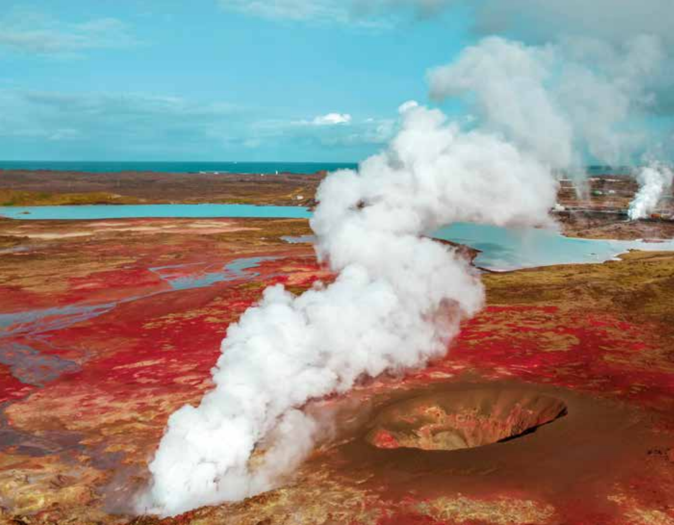
Gunnahver hot spring geyser in Iceland with its geothermal power plant.
